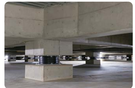
Seismic isolation structure of the new plant
