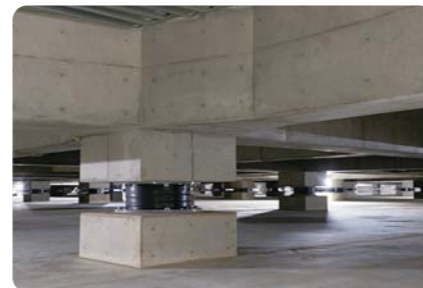
Seismic isolation structure of the new plant
